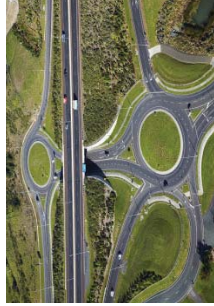
FIGURE: Exit Ramp Roundabout
